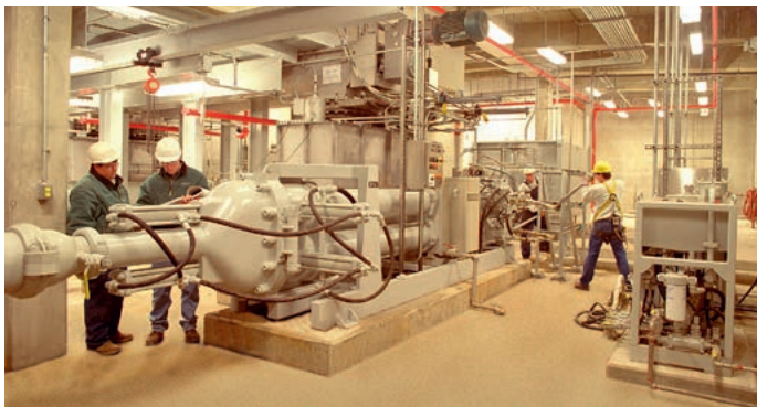
WWTP Blue Plains, Washington, D. C., USA
